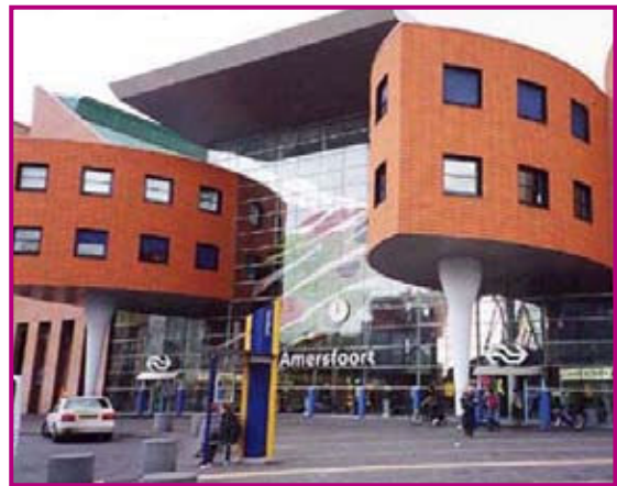
Mixed use development at Amersfoort railway station
