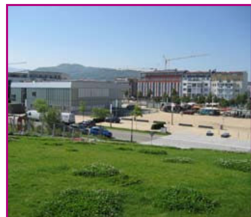
A green roof connects the sports centre with the school and the shops in Rieselfeld
